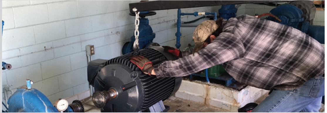
Push comes to shove as Scott and Joe get this 865 pound 60 HP motor under control.
