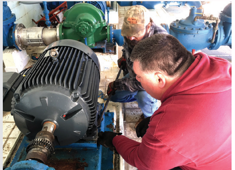
Setting up and calibrating the laser alignment tool on the pump and motor shafts.
