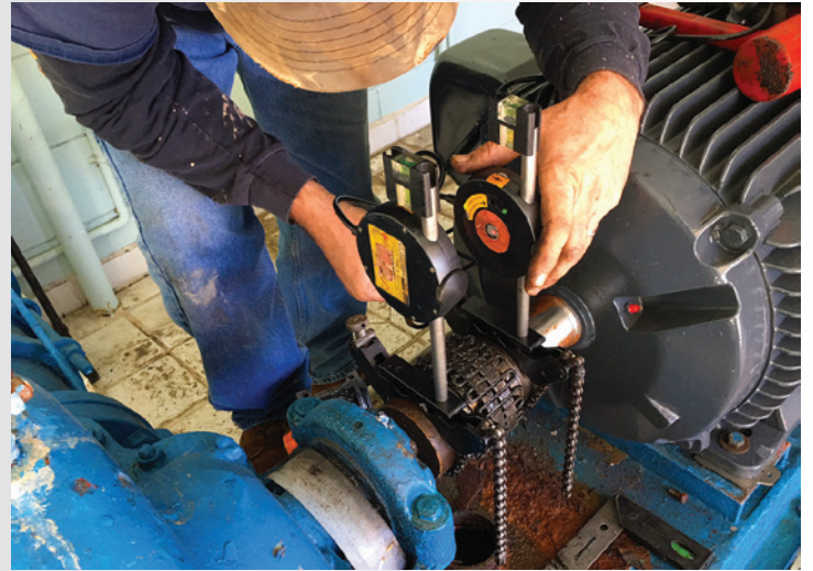
Setting up and calibrating the laser alignment tool on the pump and motor shafts.
