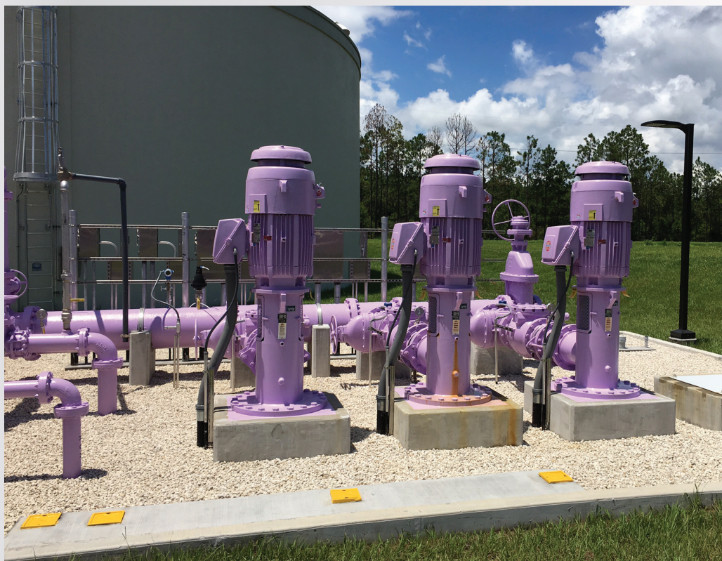
Scott Thurrott sends a photo of these 1750 GPM/125 HP, reclaimed water distribution can pumps.
