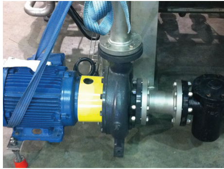
Jack Kirkwood reports a Gusher close coupled ANSI pump installation at ALLPAX Products. These pumps are being used in sterilization retorts for food processing industry and the application is superheated water.
