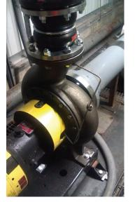
These Gusher ANSI pumps were sold to and installed at Yamaha in Newnan, Georgia. Their service is paint sludge system recirculation. They replaced vertical mount pumps. The pumps are primed via use of a foot valve.
