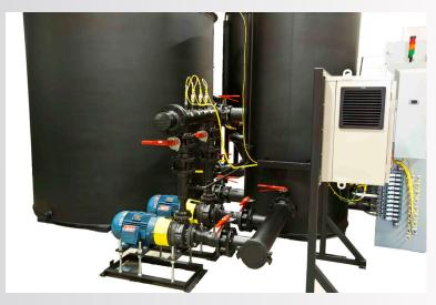
Shown is here are Gusher pumps integrated with a CoorsTek system. CoorsTek is the largest silicon and ceramic producer in the world. This system to supplies 20 grinding machines with clean water based coolant at rate of 300 GPM. The system utilizes Gusher pumps for the filter pump and the clean supply system. All of the pumps are driven with VFD controls.
