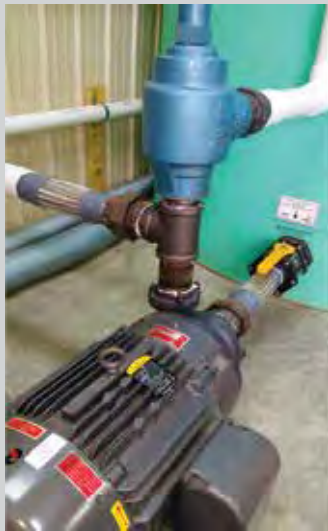
An engine dyno system equipped with a Fulflo relief valve.
