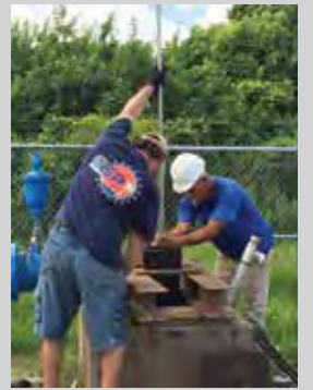
Making way for new Deming® Vertical Turbine Pumps, which feature Self-Seal design. This construction eliminates the need for packing and costly mechanical seals.
