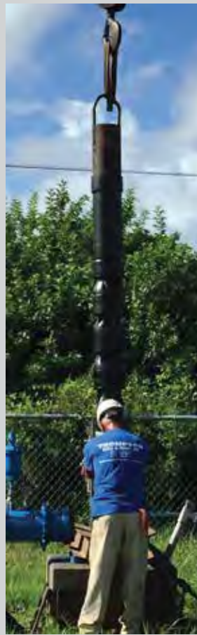
Making way for new Deming® Vertical Turbine Pumps, which feature Self-Seal design. This construction eliminates the need for packing and costly mechanical seals.
